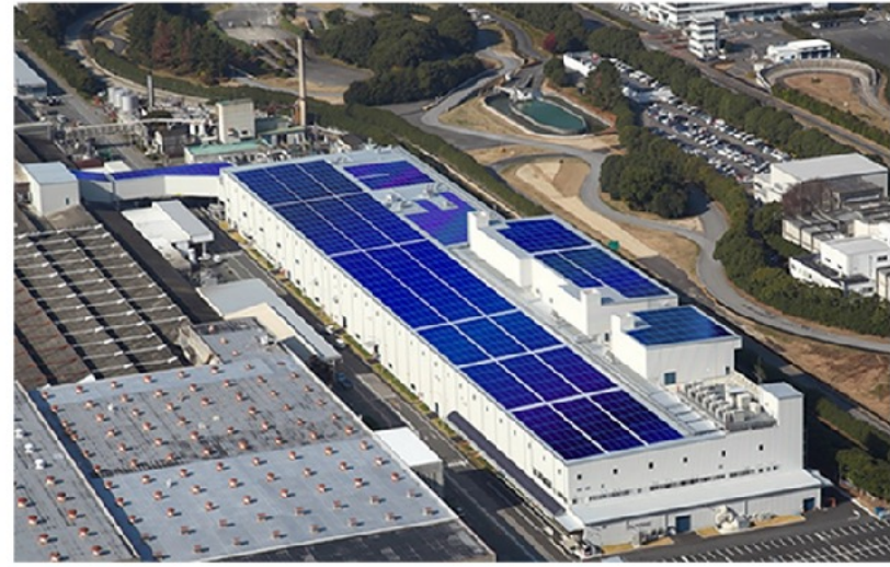
Mitsubishi built this rooftop solar-plus storage system.
